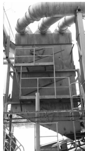
Figure 3. Industrial counterflow cooler with a capacity of 17 t/h.
