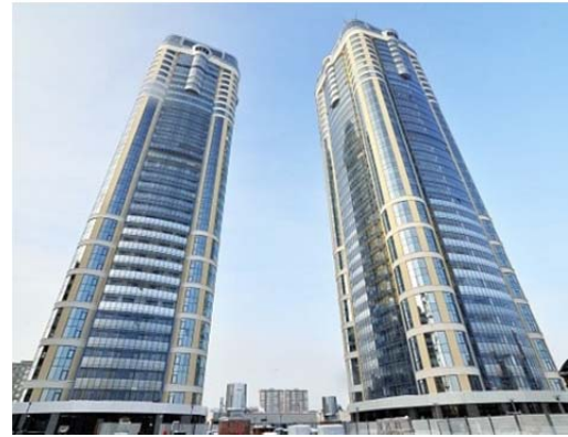
Figure 2. "Champion park" residential complex. Progress of works.
