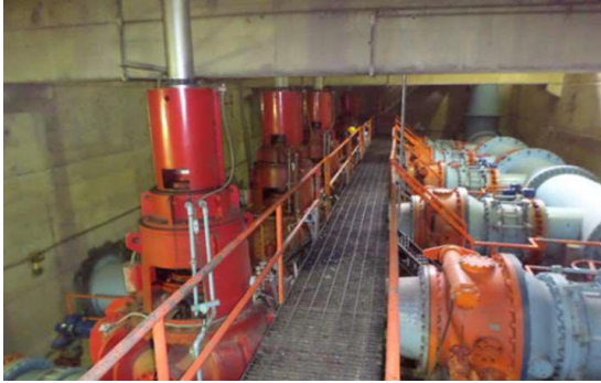
Figure 1. Parallel system of multiple pumping units
