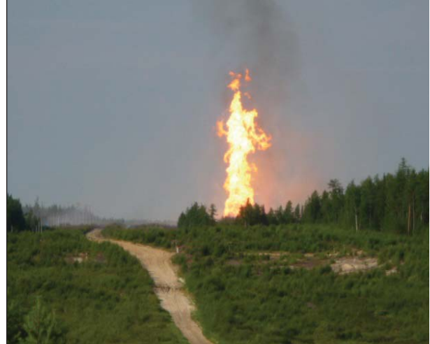
FIGURE 2. Accident due to SCC
