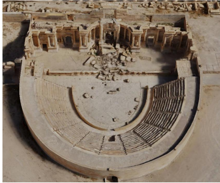
FIGURE 4. 3D model for the damaged Roman amphitheater-Palmyra city.
