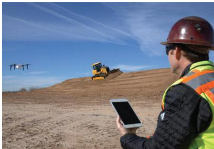
Fig. 6. Process of inspection by UAV
