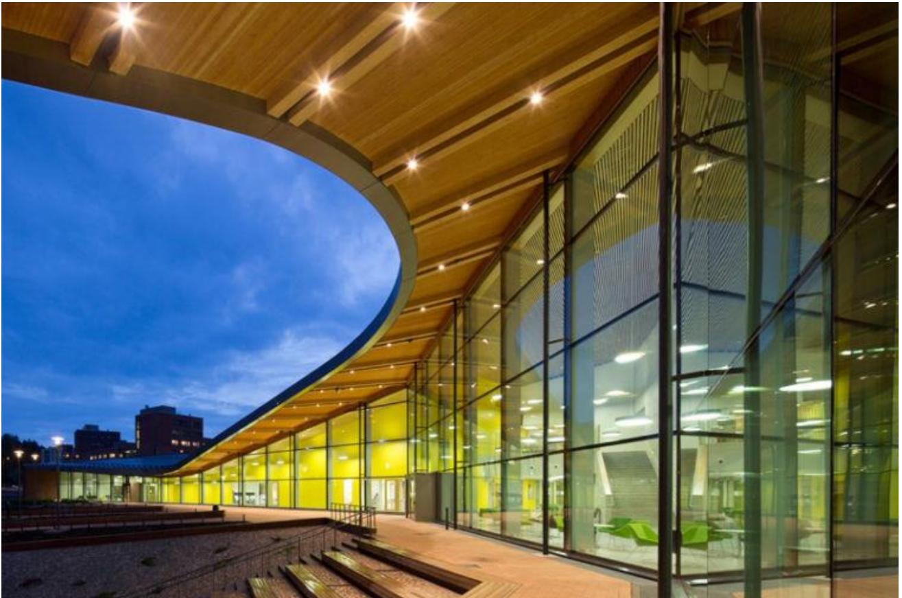
Fig. 1. The building of the «Saunalahti» school in Finland.
