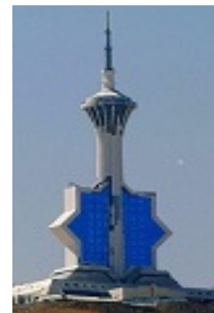
Figure 3. Television and broadcasting center "Turkmenistan", 2011.
