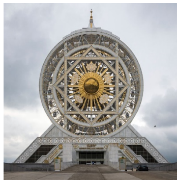
Figure 2. Cultural and entertainment center "Alem", inside the Ferris wheel, 2012.
